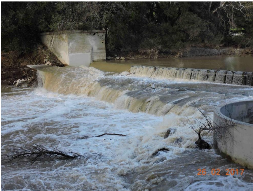
Photo 4. Metcalf Pond dam on 26 February 2017 at approximately 700 cfs, with impassable apron and lowered dam panels.
