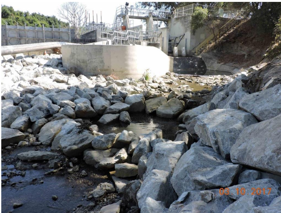
Photo 8. Boulder weir fishway construction leading to fish ladder on 3 October 2017.
