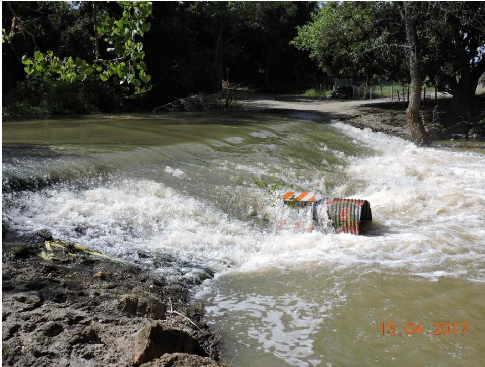
Photo 11. Singleton Road at approximately 450 cfs on 15 April 2017, impassable due to high velocity in the culverts and on the inclined apron.
