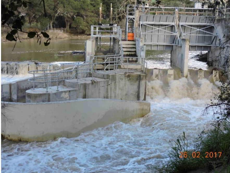
Photo 5. Metcalfe Pond radial gates and impassable (no flow) fish ladder on 26 February 2017.
