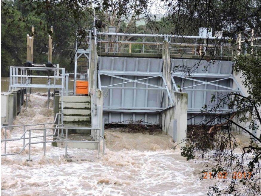
Photo 3. Metcalf Pond ladder and radial gates on 21 February 2017 at 6500+ cfs. The pond water level was high enough that even with the dam panels down there was potential passage in the fish ladder.
